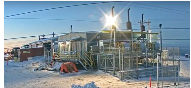
Sachs Harbour Power Plant Oct 2022
