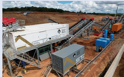
Example: Construction of Modular Process Plant
