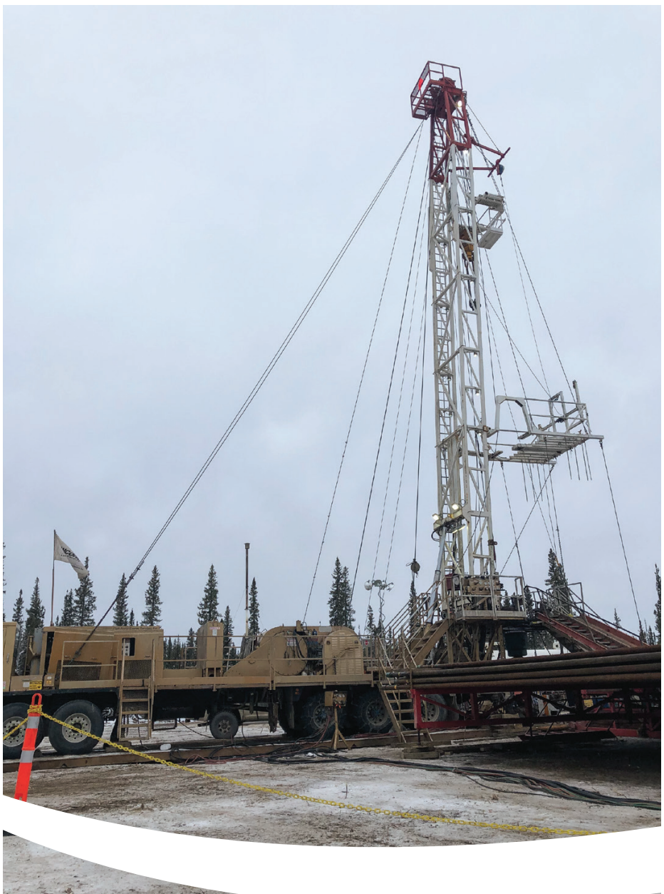
Service rig, Fort Liard area, February 2020. (Credit: OROGO)
