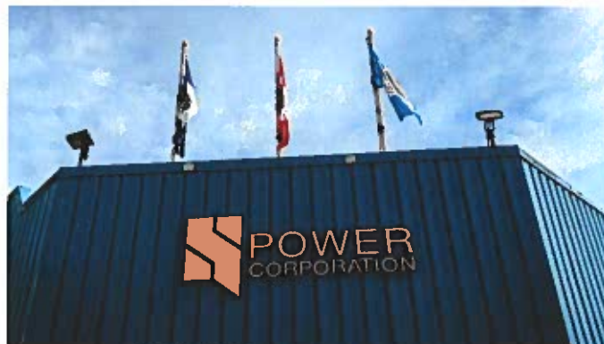
A file photo of the NWT Power Corporation building in Hay River. Ollie Williams/Cabin
