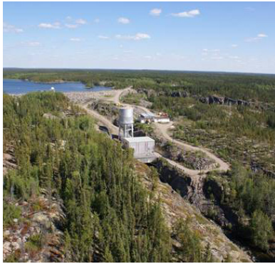
Current Taltson hydro facility
