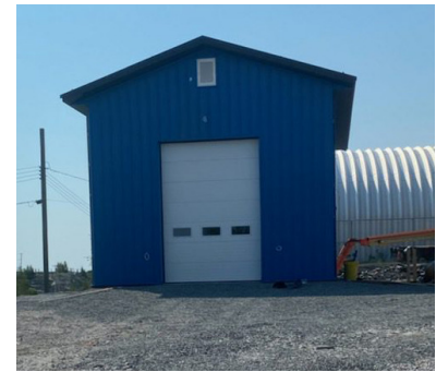
Great Slave Bottling Company's new facility
