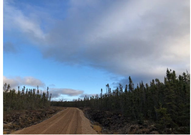
Newly constructed section of the Austin Lake Access Road in Łutselk'e.
