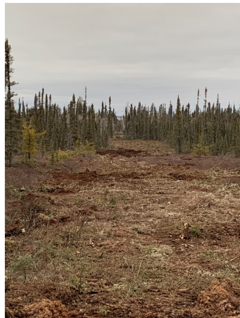
Construction on the Edzo Section of the 1.3 km Behchokò Access Trail.
