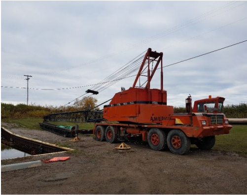
Long-boom crane and pile driver during construction at Porritt Landing Marina.
