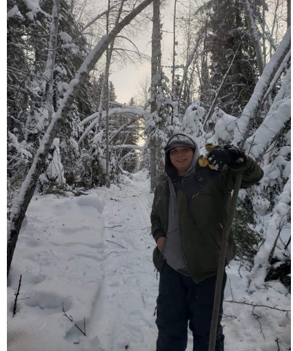
Access trails construction with chain saws in Nahanni Butte.
