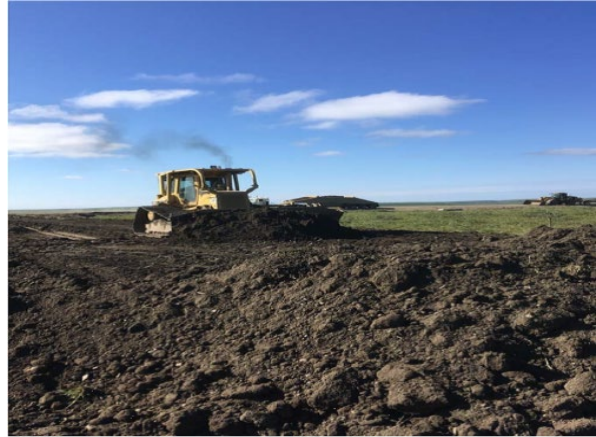
Heavy Equipment Operator operating a bulldozer during Husky Lakes Trail construction.
