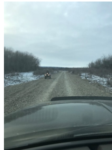
Happy's Landing Boat Launch Access Road after application of aggregate.
