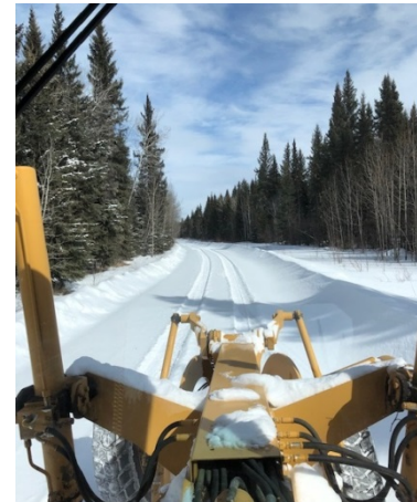
Grader operations on the Grande de Tour Winter Road in Fort Smith.
