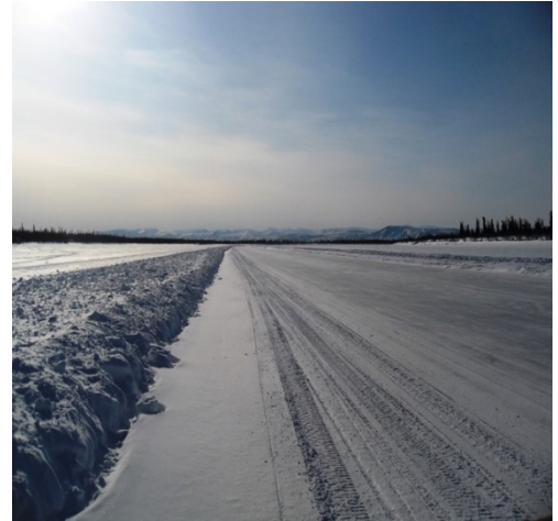
A view along the 80 km Fort McPherson section of the Peel River Ice Road constructed from Fort McPherson to the Esau Creek.
