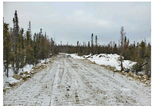
Duck Pond Access Road in Gamètì after the conclusion of 2020-21 construction.
