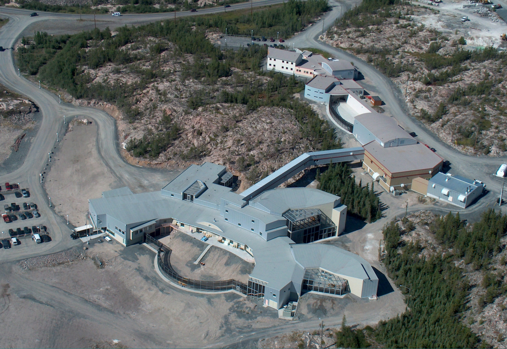
North Slave Correctional Facility
