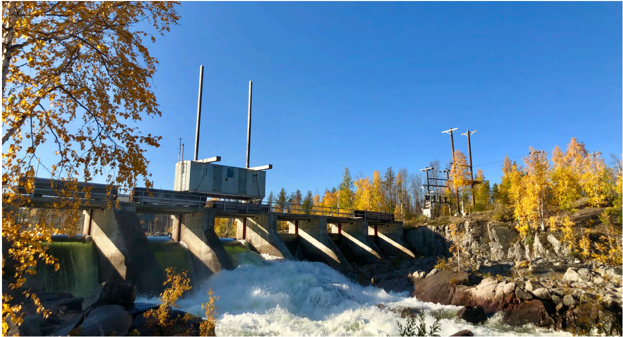
Upgrades to Unit 1 of the Snare facility were completed in the summer of 2021.
