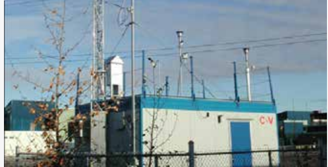
Air Quality Monitoring Station. (GNWT)
