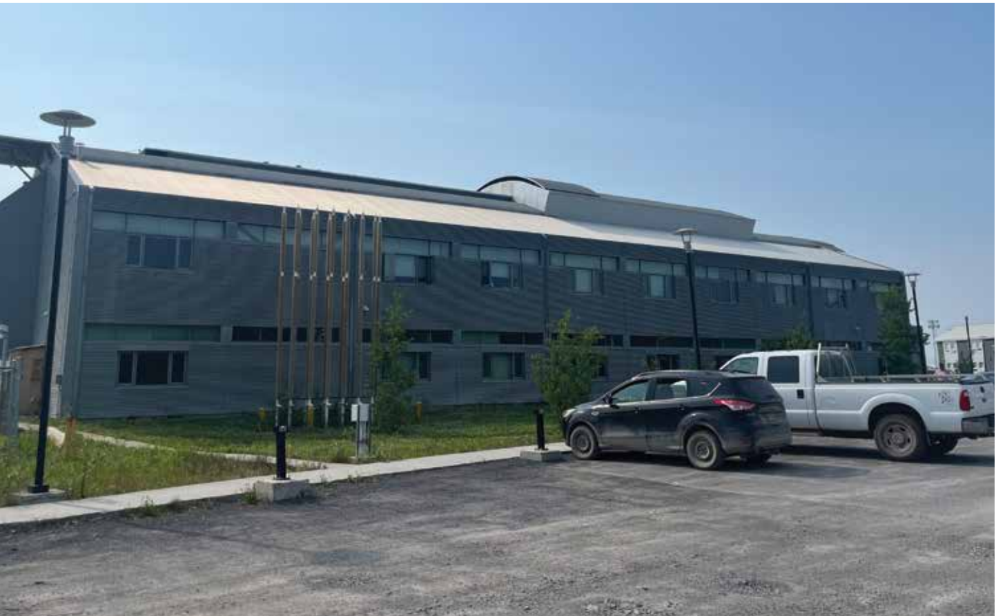
Inuvik's Aurora College campus and student residence has received LED lighting and a Direct Digital Control system through CARF.
