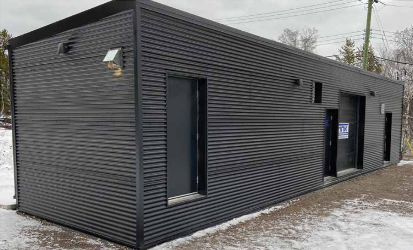
Yellowknife's Sissons Court district heating system project was completed in 2022.
