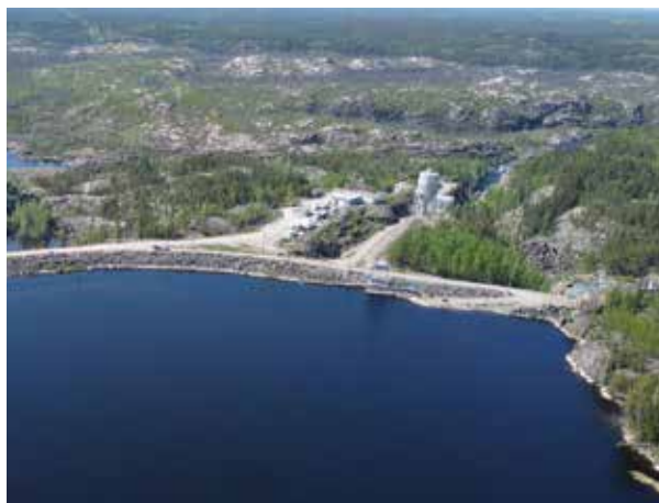
New work camp (left) to house workers upgrading the Taltson Hydro facility (right).
