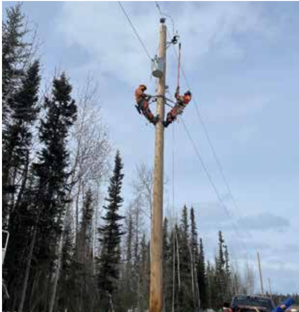
The arrival of new housing units in Jean Marie River required installation of new power poles and the replacement of the transformer substation. This major project was completed in fewer hours than budgeted because of great teamwork and widespread community cooperation and support
