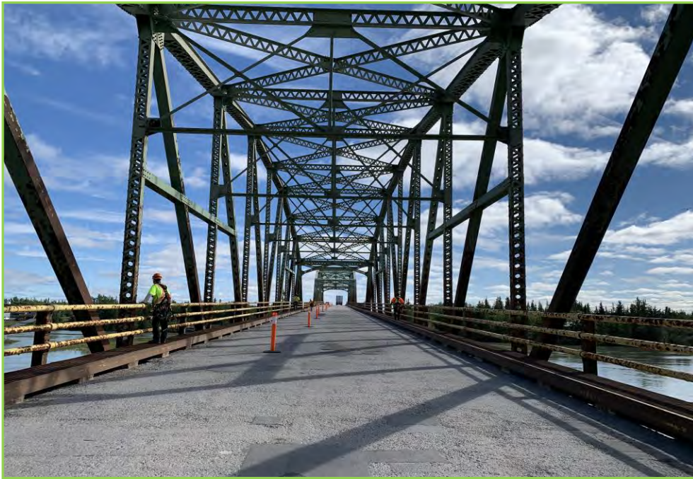
Photo 11 – General View of the Span 1
