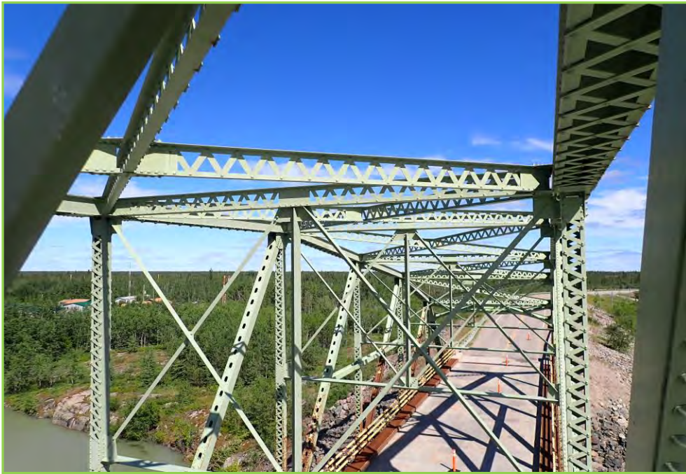
Photo 085 – Top Chord and Bracings are in Good Condition, Span 4
