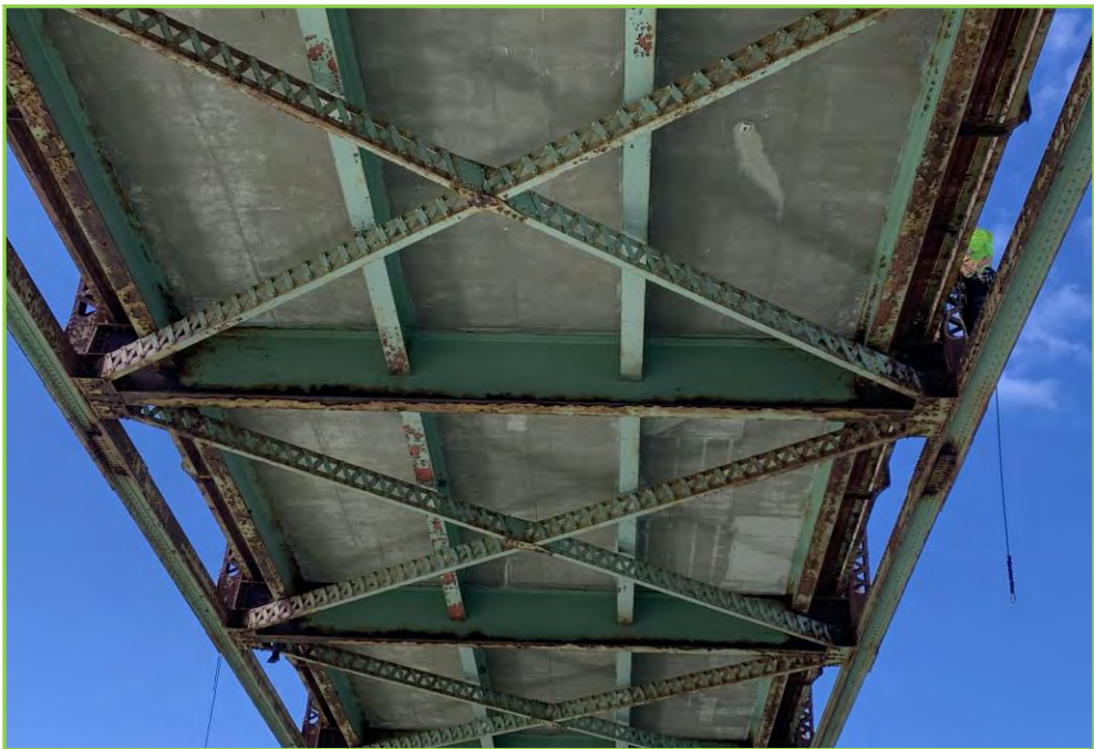
Photo 039 – Underside of Span1, Stringers and lateral Bracings, Typical
