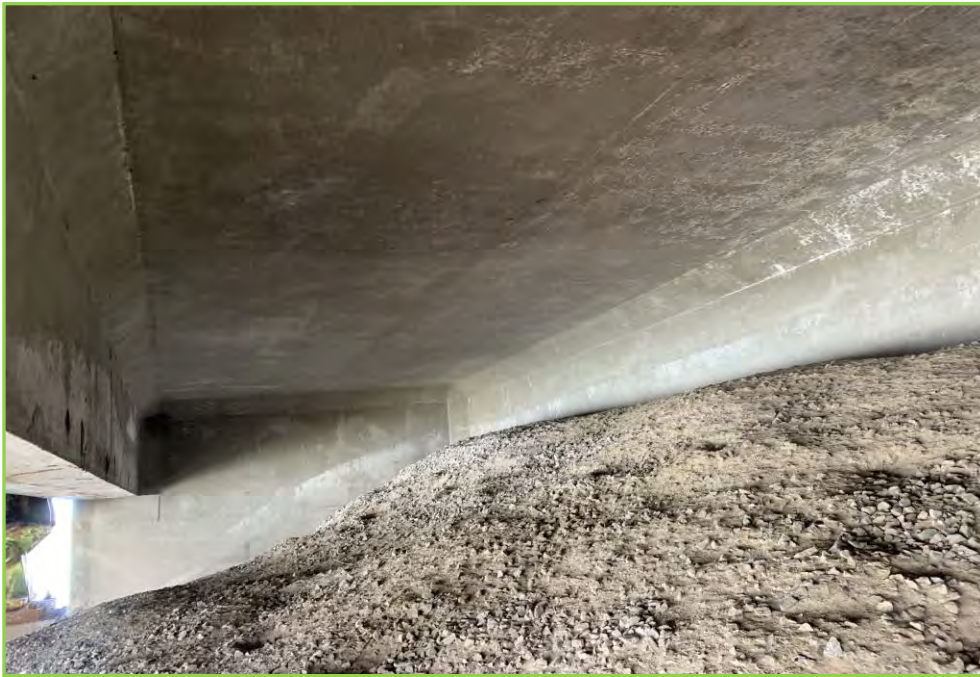
Photo 077 – Roof Slab at Abutment 2
