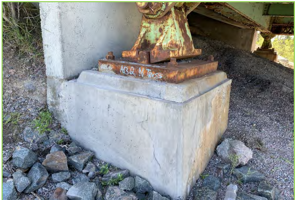
Photo 074 – Bearing Seat at Northeast, Abutment 2.
