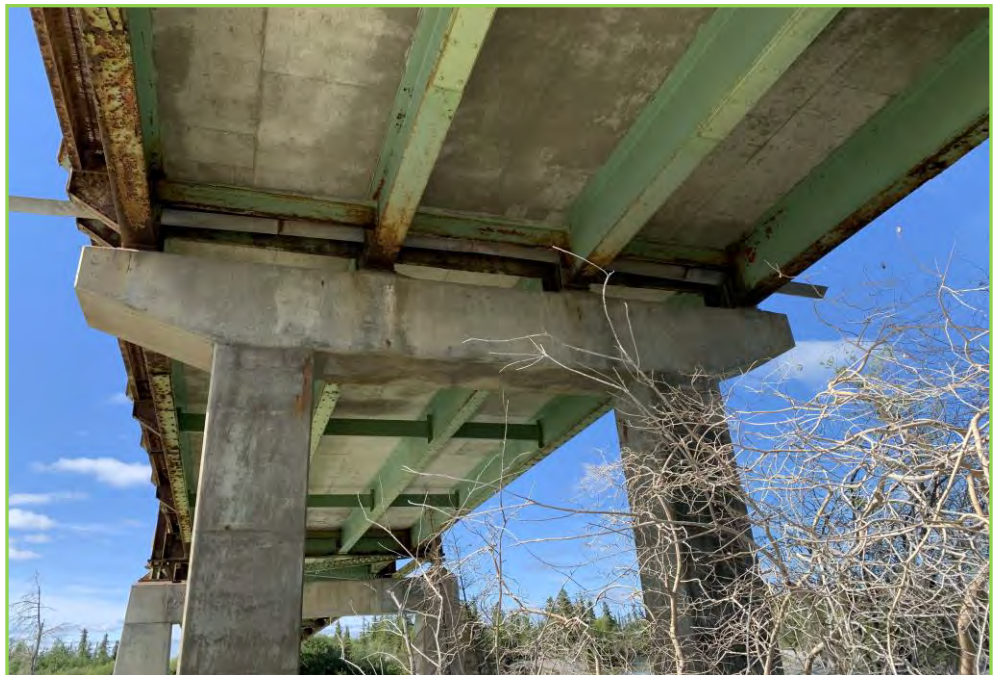
Photo 050 – Pier 2 Looking West.
