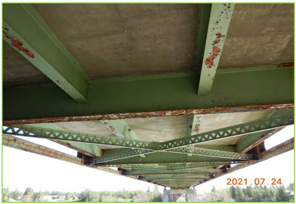
Photo 040 – Stringers at Span 1, Typical in Good Condition
