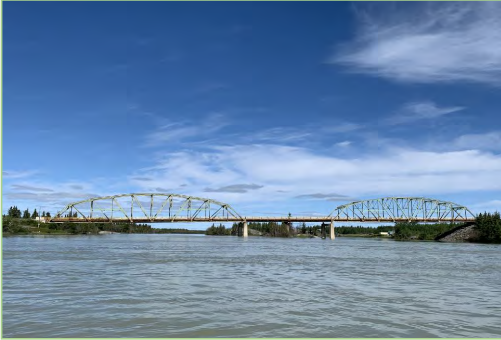
Photo 1- Elevation View Looking North
