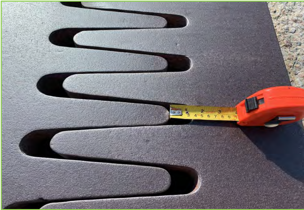
Photo 029 – Deck Joint at Abutment 2
