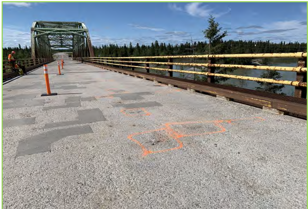
Photo 12 – Concrete Deck patching at Span 3
