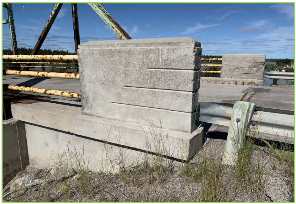
Photo 070 – Concrete Parapet and Wingwall at Southeast, Abutment 2
