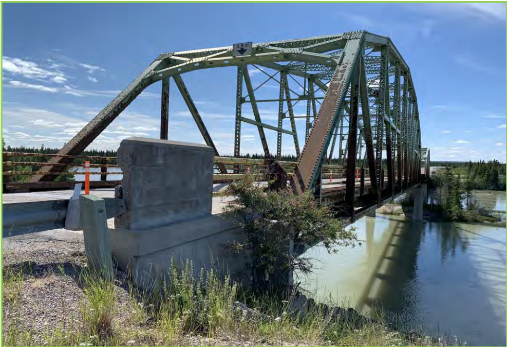
Photo 068 – Concrete Parapet and Wingwall at Northeast, Abutment 2
