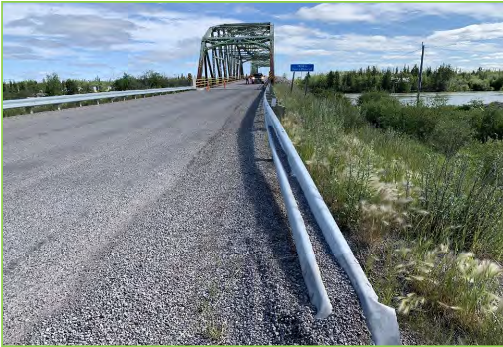
Photo 081 – Turndown End Treatment at Southwest, Typical in Good Condition
