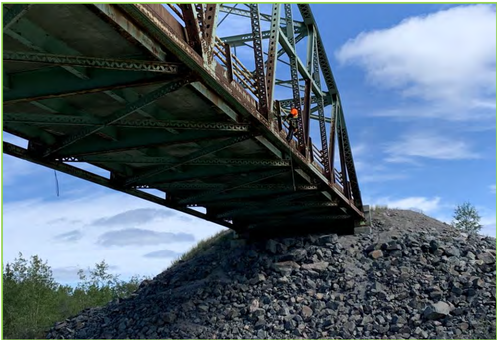
Photo 069 – Riprap Slope Protection at Abutment 2
