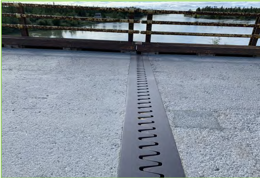
Photo 027 – Deck Joint at Pier 2
