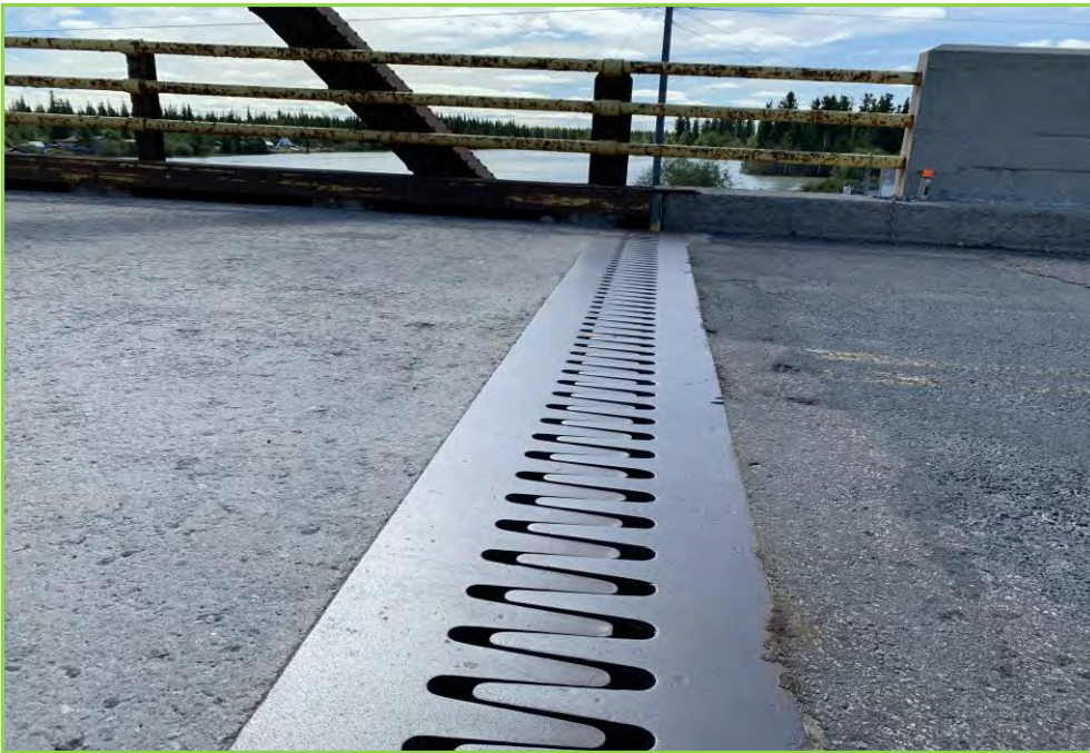
Photo 025 – Deck Joint at Abutment1
