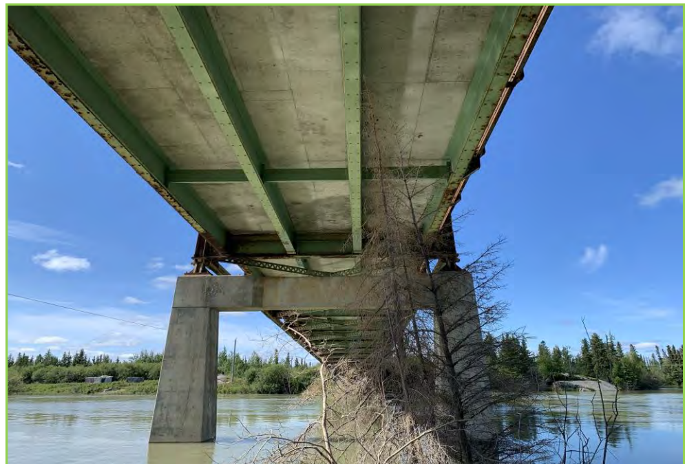
Photo 022 – Deck Soffit at Span 3
