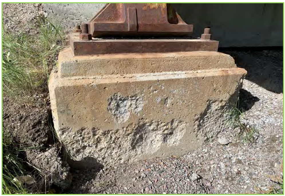
Photo 4 – Abutment seat at Abut 1, Southwest, Minor Concrete Spall
