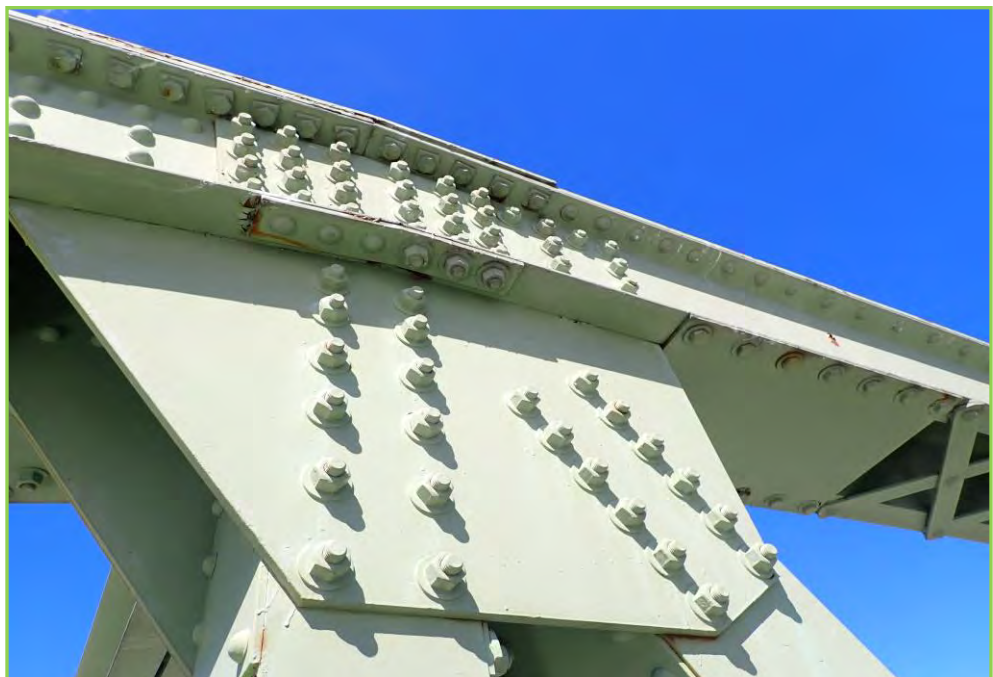
Photo 086 – Connection of the top Chord and Vertical/Diagonal, Typical Good Condition, Span 4
