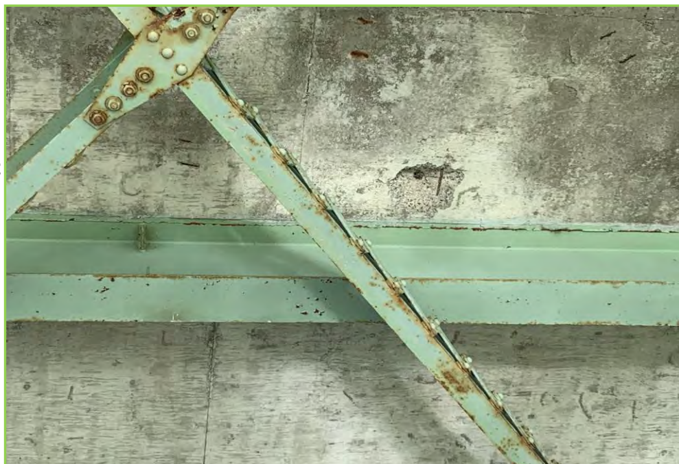
Photo 024 – Deck Soffit Small at Span 1
