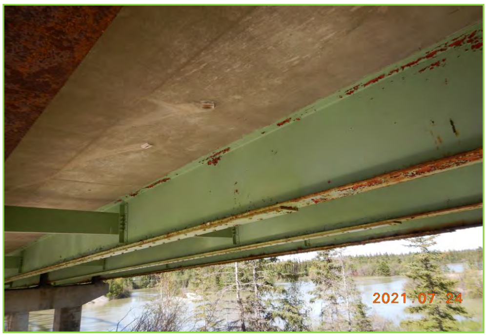
Photo 066 – Interior Girder at Span 3, General in Good Condition
