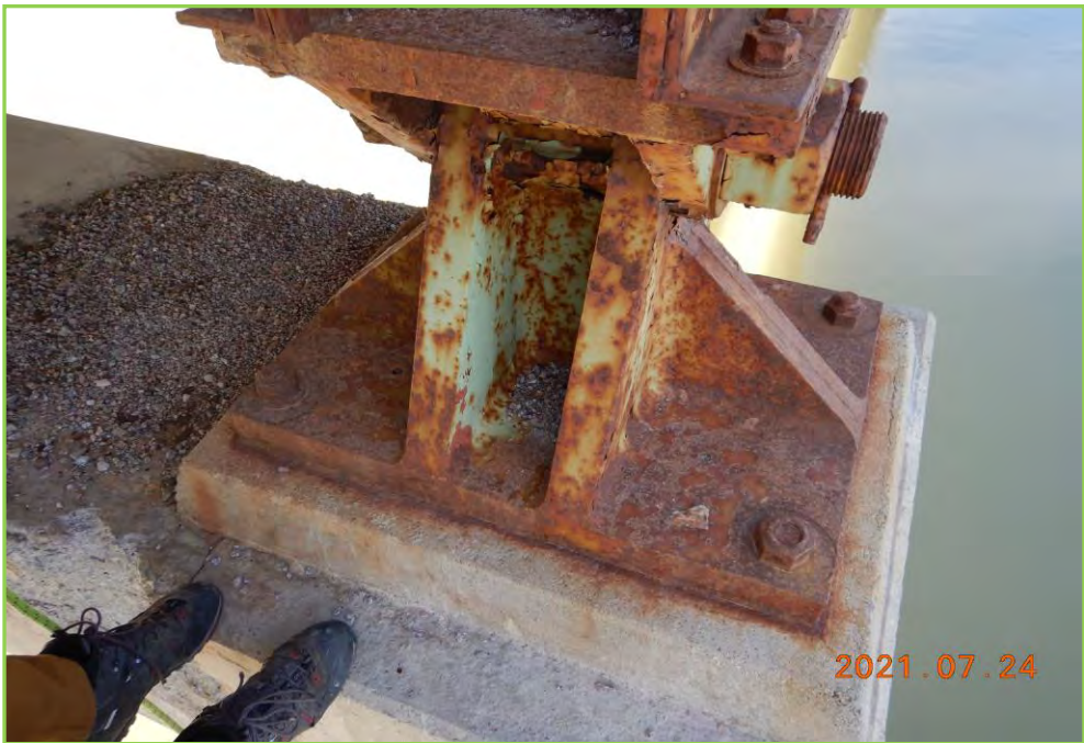
Photo 047 – Bearing at Pier 1, Light Corrosion
