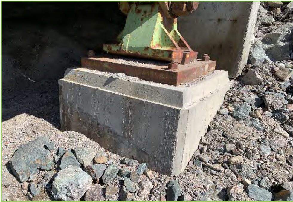
Photo 073 – Bearing Seat at Southeast, Abutment 2.
