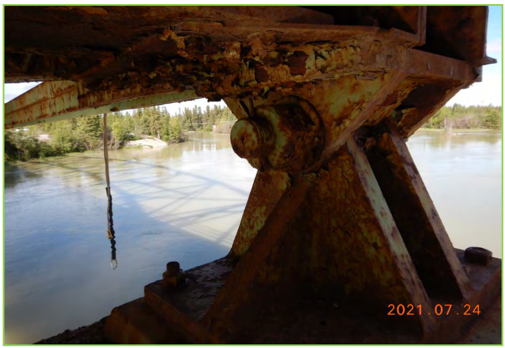
Photo 048 – Rock Bearing at Pier 1
