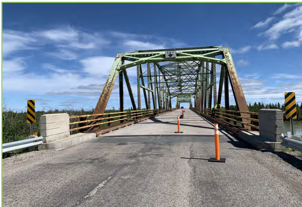
Photo 6 – Approach at Abutment 1
