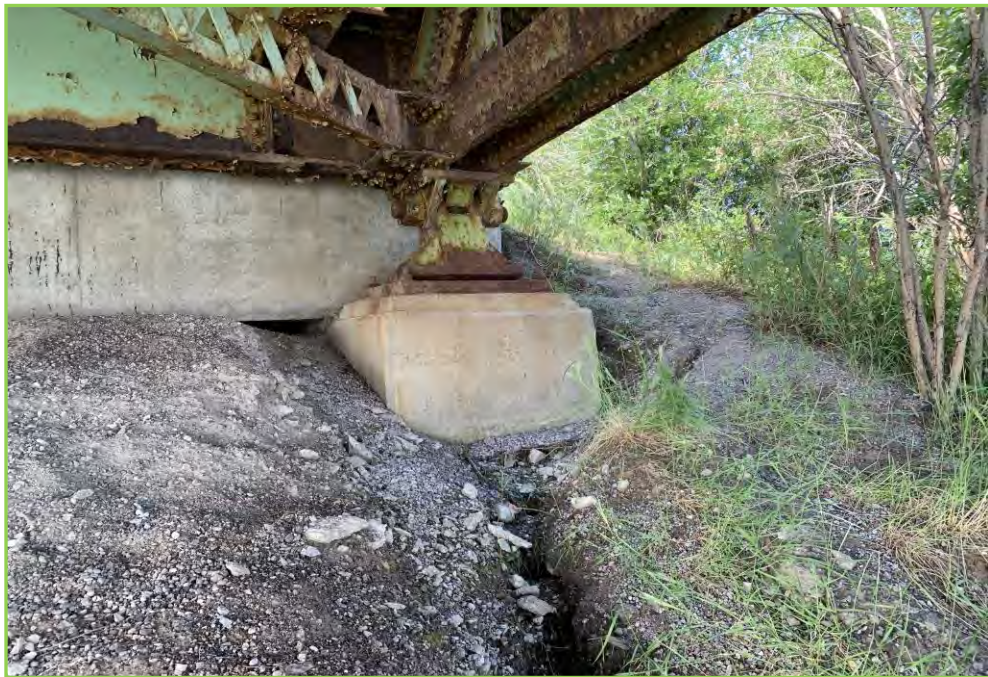
Photo 5 – Bearing Seat at Abutment 2, Northwest, Gully at the Headslope
