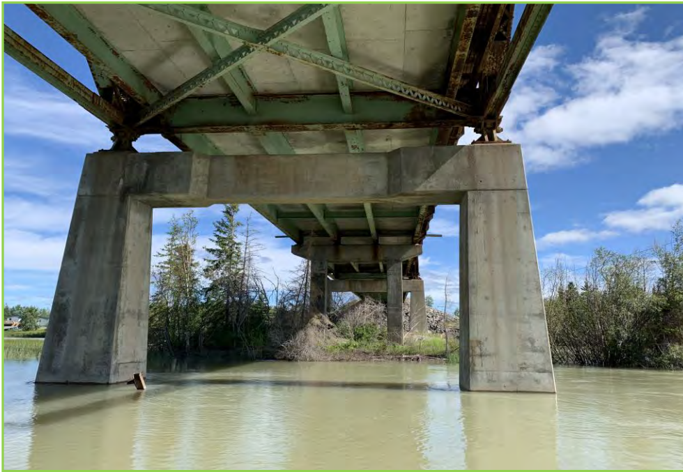
Photo 045 – Pier 1 Looking East, In Fair Condition
