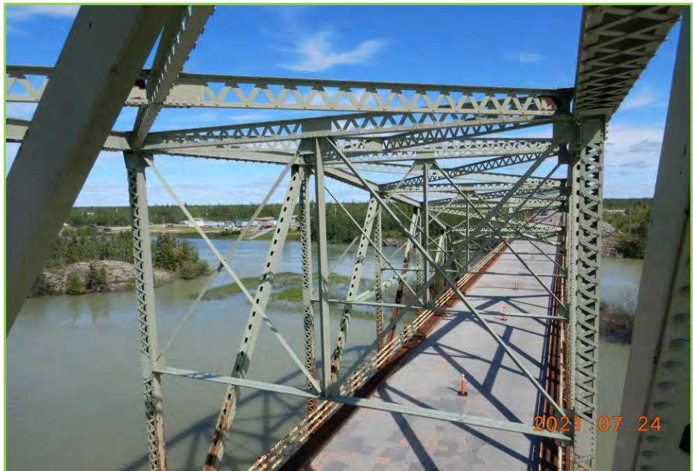
Photo 082 – Top Chord and Bracings are in Good Condition, Span 1
