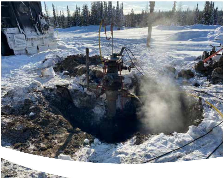
Hydro-cutting a wellhead, Cameron Hills, March 2023. (Credit: OROGO)
