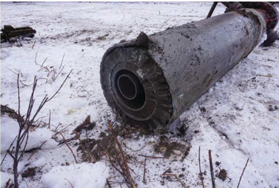
Wellhead and casing removed during the abandonment process, Cameron Hills, February 2024. (OROGO)
