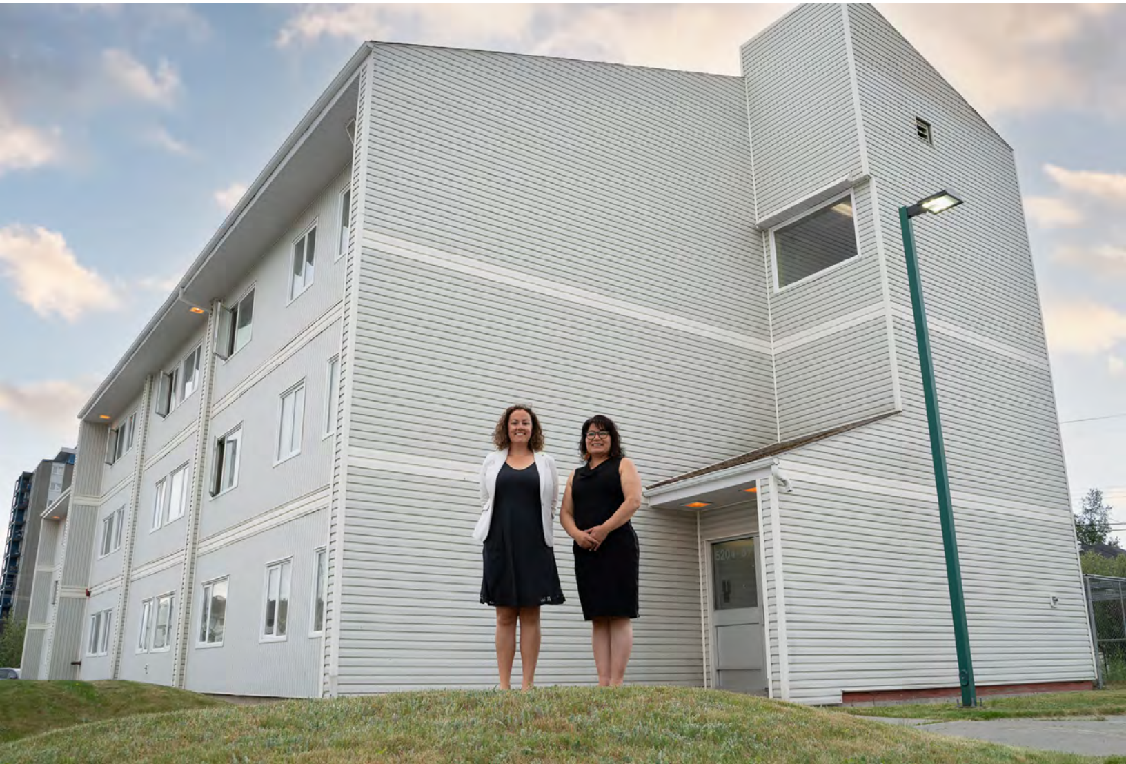
Aspen Apartments in Yellowknife, NWT Photo Credit: Housing NWT
